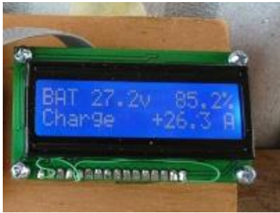
Fig. 4: Battery monitoring display
